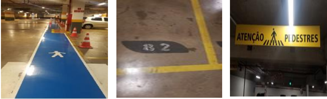
Figure 4.35: Parking space in companies A and B with signs that ease movement
