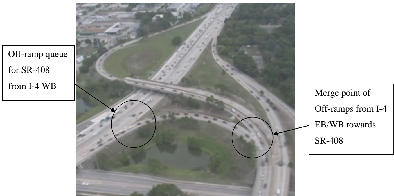
Figure 5.7 Snapshot of the bottleneck located at the off-ramp to SR-408 from I-4 WB
