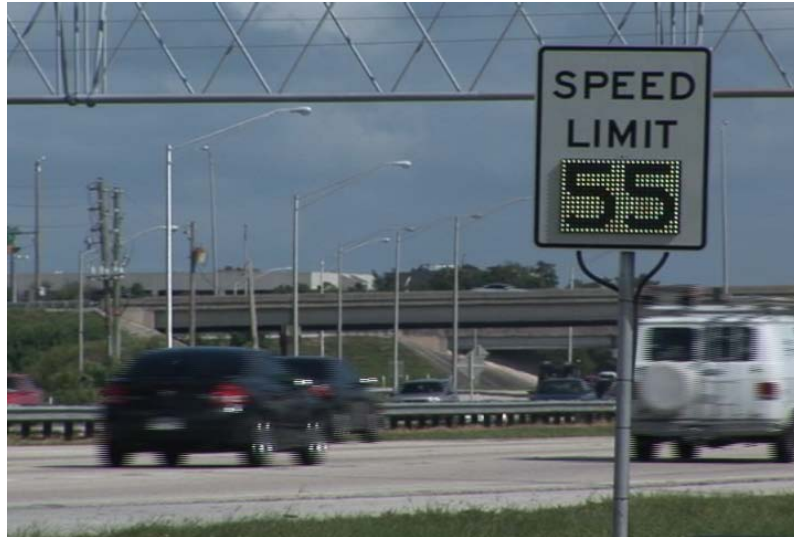
Figure A.4 Variable Speed Limit Sign on I-4 in Orlando, FL
